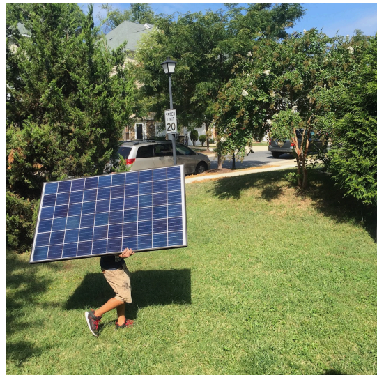
Solar panels being installed on the author’s roof.
